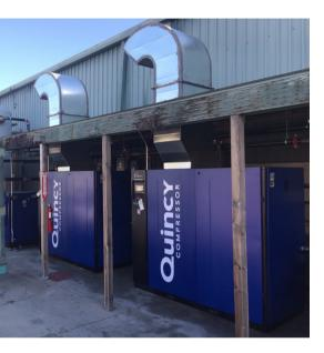
We ordered, delivered and installed the equipment by November 2021. We provided a lead/lag solution with twin QGV-75s, which will provide adequate CFM with the expansion in mind. It will also reduce overall energy, installation and purchase cost compared to Atlas Copco.
